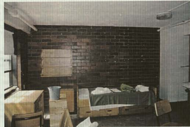
Fig. A40 Electrical & Teledata Rewiring Student Rooms
