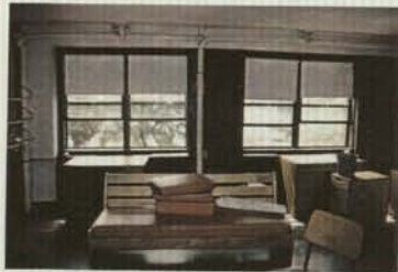
Fig. A32 Existing Heating Student Rooms
