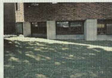
Fig. A3 Concrete at the building's foundation
