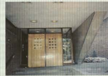
Fig. A4 Triangular-shaped pier supporting north entry
