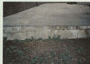
Fig. A19 above South terrace bluestone pavers
