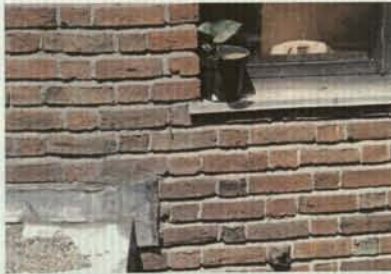
Fig. A7 above Section of south elevation exhibiting both original gray mortar (upper left section) and discolored tan mortar (lower right section)
