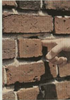
Fig. A7 above Section of south elevation exhibiting both original gray mortar (upper left section) and discolored tan mortar (lower right section)
