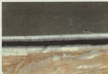
Fig. A31 Paint stratigraphy from door casing in Room 206 (substrate at bottom of photo)
