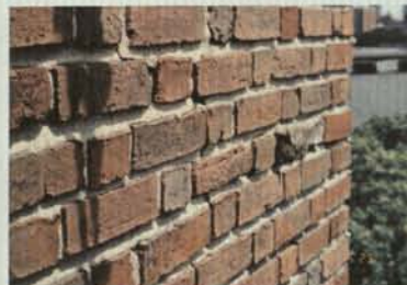
Fig. A6 Brick mortar joints
