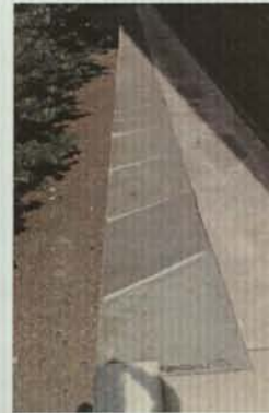
Fig. 70 Bluestone North Terrace wall cap
