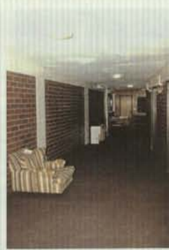
Fig. 88 Structural Tile in corridor
