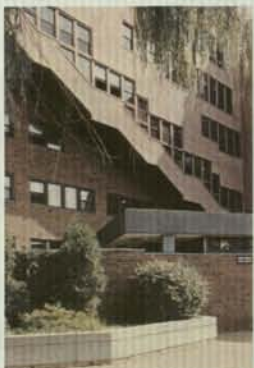
Fig. 125 North facade detail w/ cascading single-glazed windows & insulated windows below
