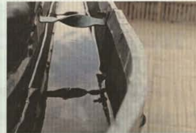
Fig. 114 above Ponding water in gutter Level "D"
