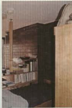
Fig. 87 Structural Tile in student room
