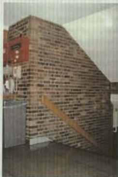
Fig. 101 Newer oak rail at main lobby stair
