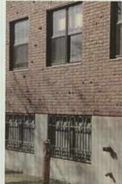
Fig. 92 Basement window grates
