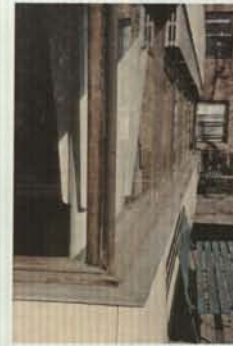
Fig. 128 Wood windows at Pavilion upper level
