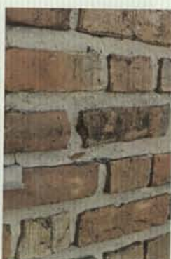
Fig. 78 South-West corner brick detail
