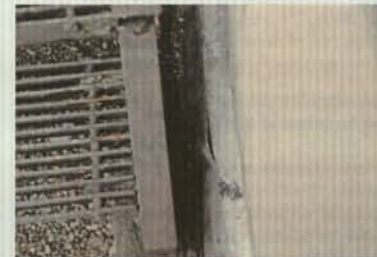
Fig. 116 Open base flashing Level "F"
