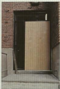
Fig. 123 New flush door at stair #4
