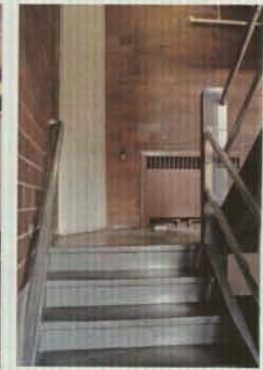
Fig. 94 Fire stair #1 railing
