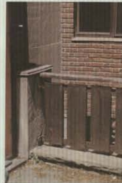
Fig. 95 Wood railing at North side of Pavilion
