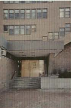
Fig. 85 Slate panels at North Entry
