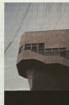
Fig. 76 Concrete support for cantilevered north stair
