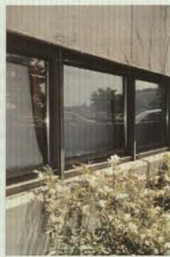
Fig. 82 Moon Garden Pavilion limestone and aluminum replacement windows
