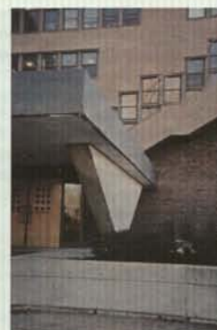
Fig. 75A North Entry Canopy w/ triangular concrete support
