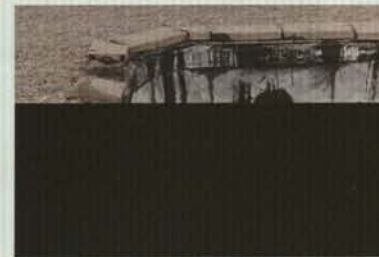
Fig. 112 above Ballast paver deterioration asphaltic mastic patching Level "A1"
