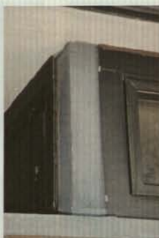
Fig. 131 Corner window condition at manager's office
