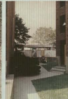
Fig. 74 Loading Dock - South Facade
