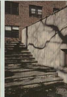
Fig. 71 Bluestone Steps and gravel landings at Moon Garden Pavilion
