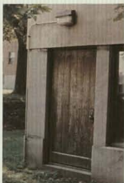
Fig. 122 Staved oak door at Pavilion lower level
