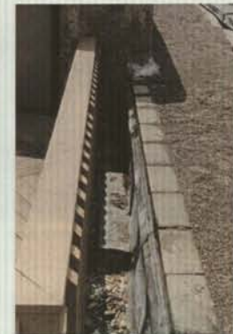
Fig. 112 above Ballast paver deterioration asphaltic mastic patching Level "A1"
