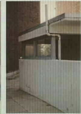
Fig. 75 Loading Dock - East Facade
