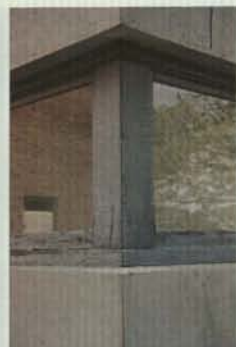
Fig. 132 Corner window at loading dock
