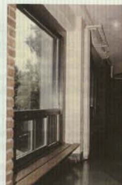
Fig. 99 Bench/convector cover at 1st floor lounge
