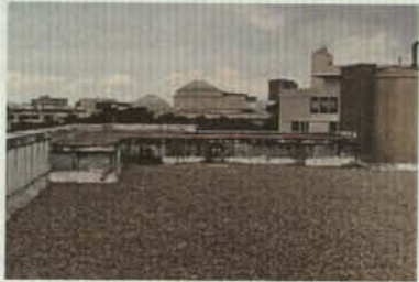
Fig. 110 left Decking supports Level "A"
