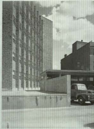
Fig. 46 View from Northwest rooms and loading dock (MIT archive - c. 1952)
