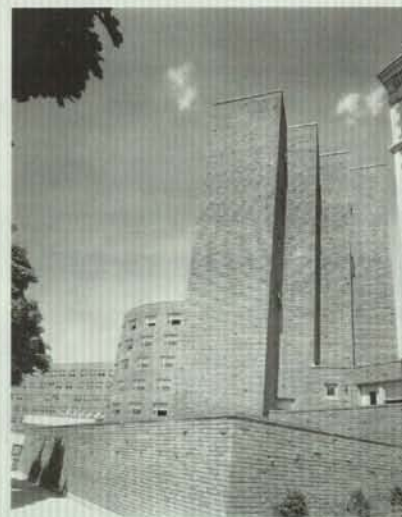
Fig. 42 East elevations, Southeast corner (ESTO - 1949)
