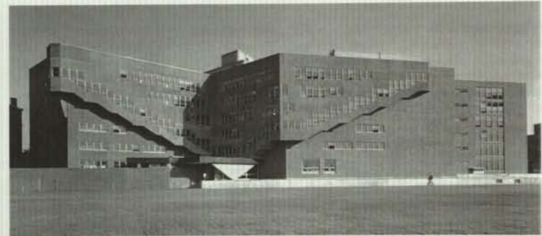
Fig. 12 North elevation (ESTO - 1949)
