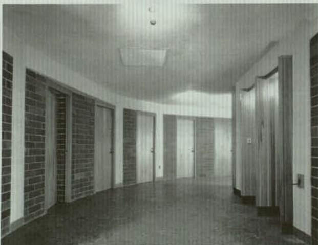
Fig. 55 Typical upper level hallway (ESTO - 1949)
