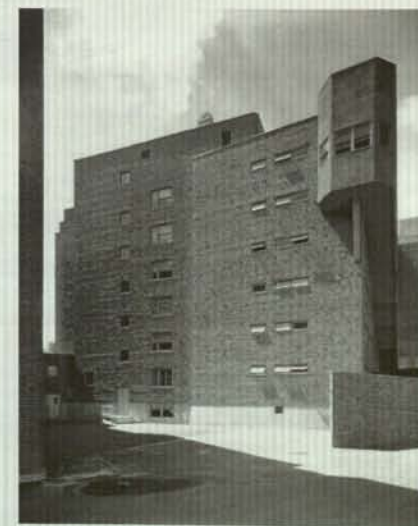
Fig. 43 East elevation, Northeast corner (ESTO - 1949) Note absence of site walls and landscaping
