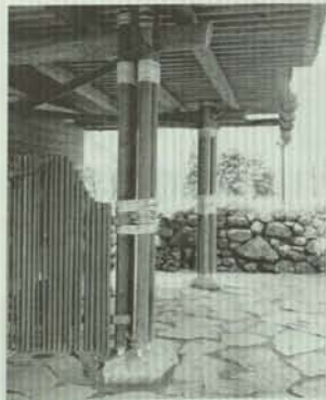
Fig. 15 Villa Mairea Exterior canopy support
