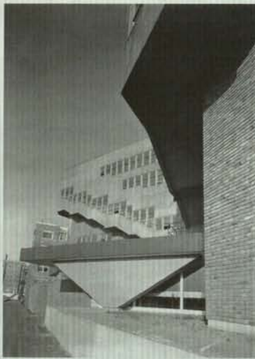
Fig. 45 View from Northwest showing Entry Pavilion and original location of Amherst Alley (ESTO - 1949)
